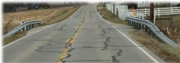
Non-Standard guardrail end treatments that are in need of upgrades
