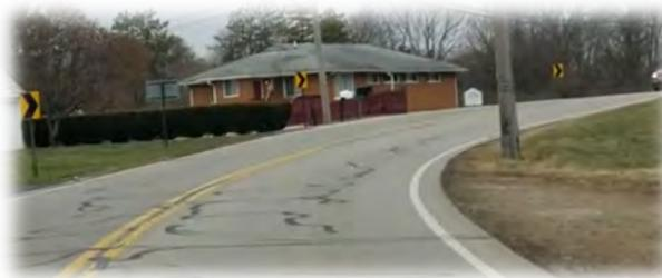
Utility pole on curved section of roadway that has been struck as it is about 3 to 4 feet from the roadway edge
