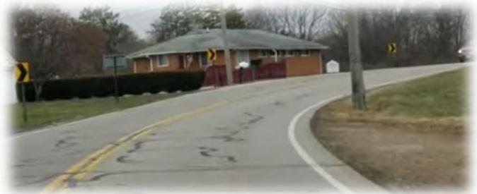
Utility pole on curved section of roadway that has been struck as it is about 3 to 4 feet from the roadway edge
