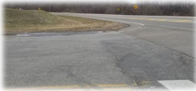
Limited sight distance at Restoration Park Drive looking northward for southbound traffic that is caused from the earth levee
